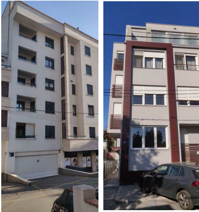
Figure 4 The newly built buildings on the site of Borisavljević's demolished houses at 35 Gvozdićeva Street and 1 Tetovska Street.
